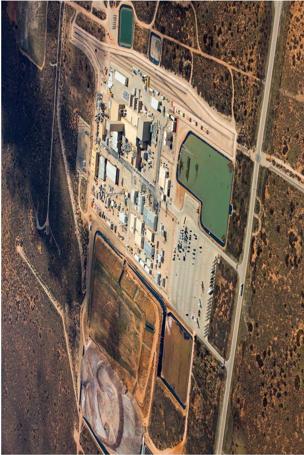
Figure B4-1 Aerial Photograph of the Waste Isolation Pilot Plant
